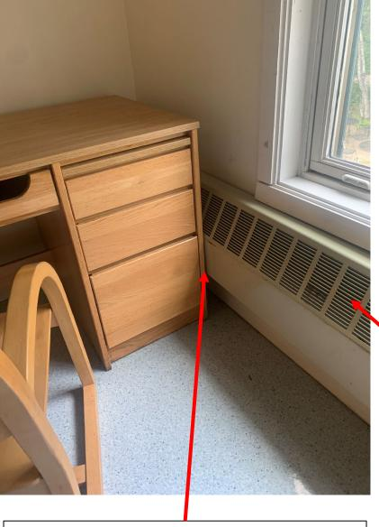
This desk is hampering a small amount of the airflow because it is tight to the heater. If this is the only blockage for this room, most likely not an issue.
