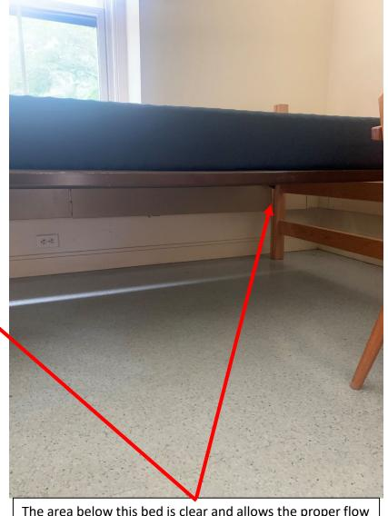
The area below this bed is clear and allows the proper flow of air through the heater. The bed appears to be touching the heater, and a bedspread can be covering up the open slats on the heater face. Pulling the bed away from the heater a few inches to keep the slats free for air movement is advised. Also, do not clutter the area below the bed with boxes or storage bins.
